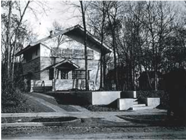
Charles Wiethoff House, Minneapolis Photo: Northwest Architectural Archives
